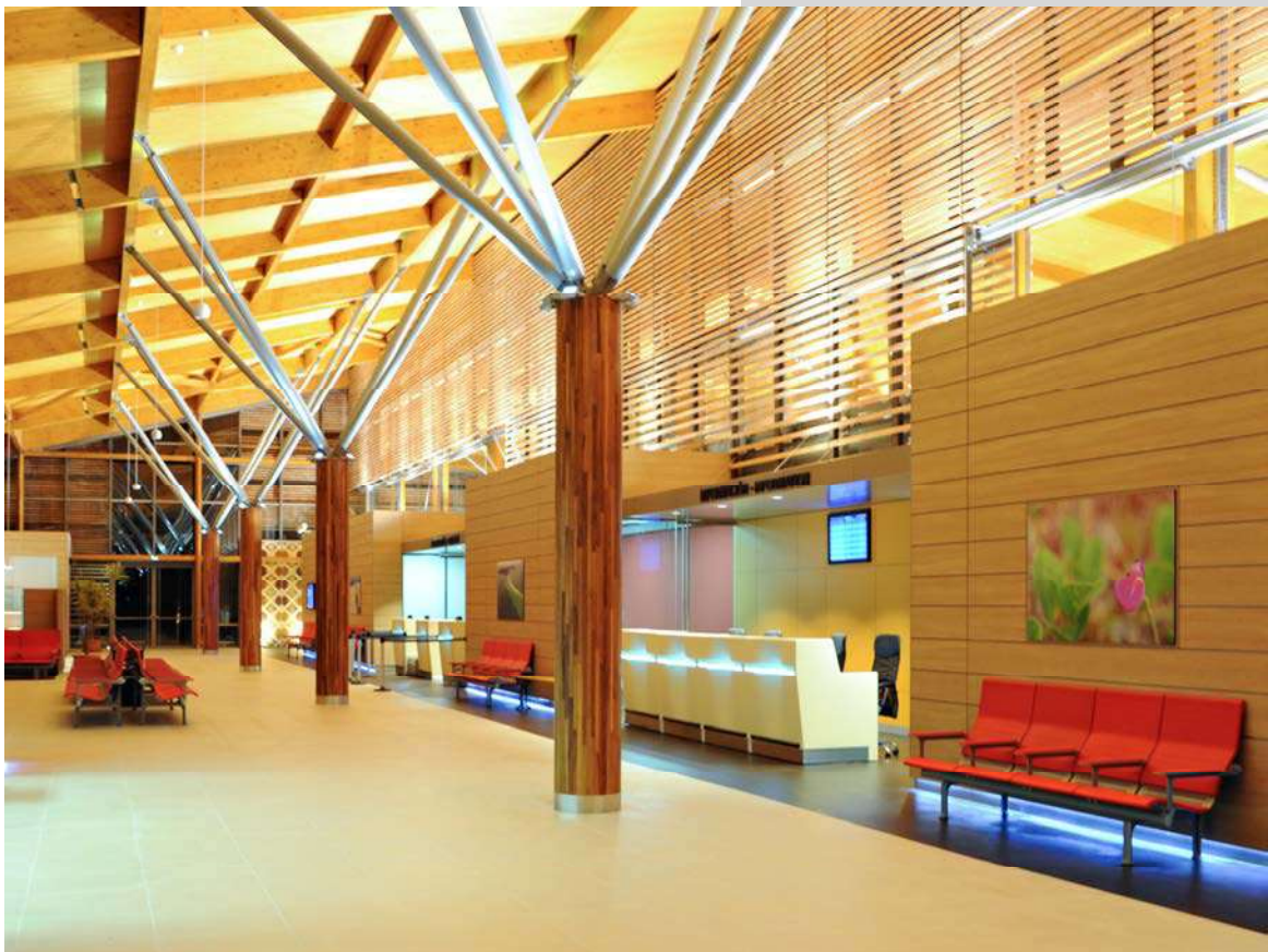
Corisco island (Equatorial Guinea) Airport Terminal Glulam structure and Sapisol® Iroko glulam round posts with Résix® connections
