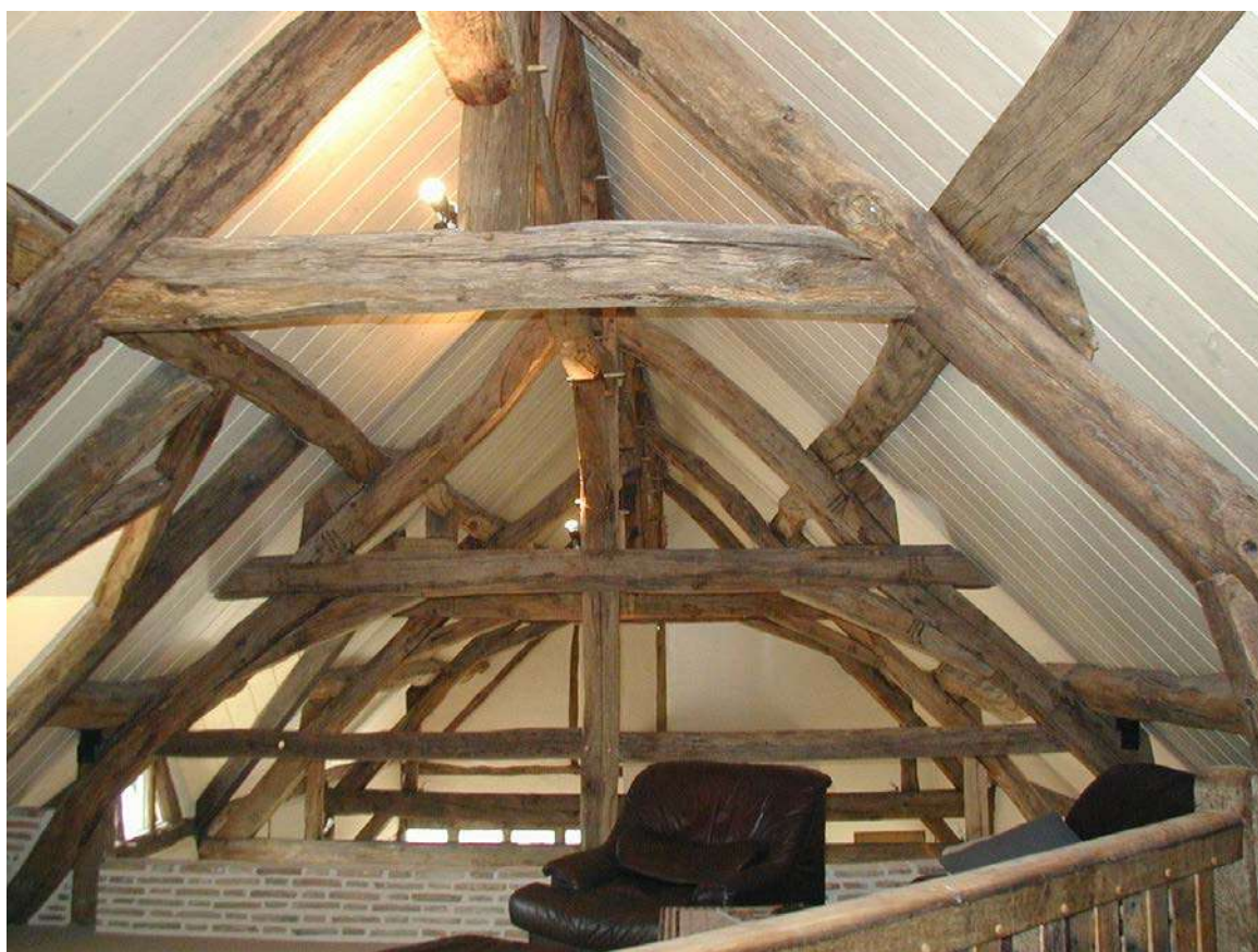
Jouy-le-Potier (France) Sapisol® roofing
