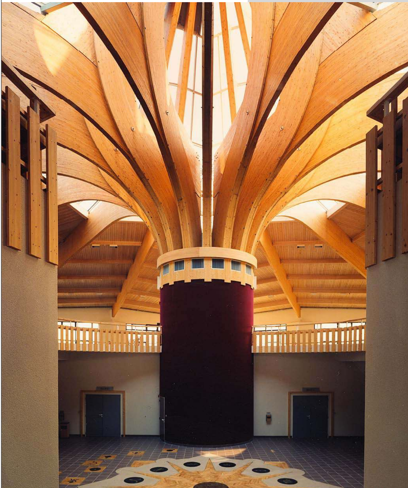
Micropolis Besançon (France) Convention Center 80m in diameter, 2m high beams
