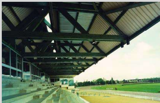
Cabourg (France) Overhanging roof at a racecourse
