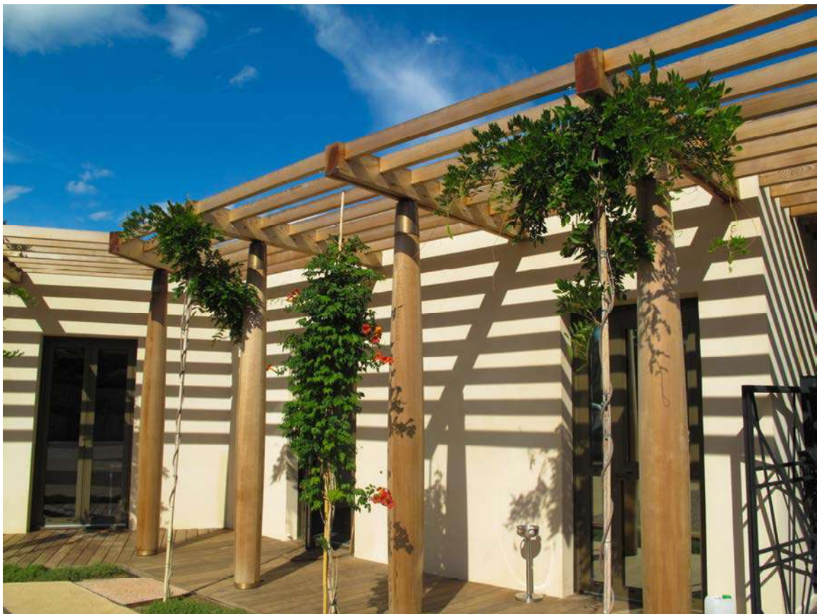
Antibes cap (France) Pergola Glulam fusiform poles with Résix® connections - Red Cedar
