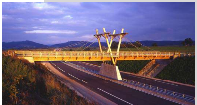
Highway bridge (designed for road traffic) Douglas fir structure with Résix® connections
