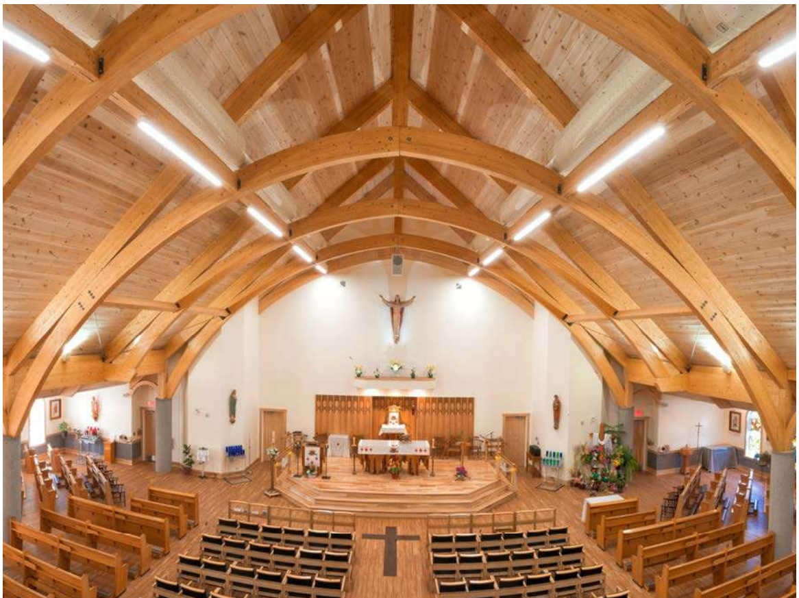
Quebec (Canada) Church Curved spruce glulam trusses
