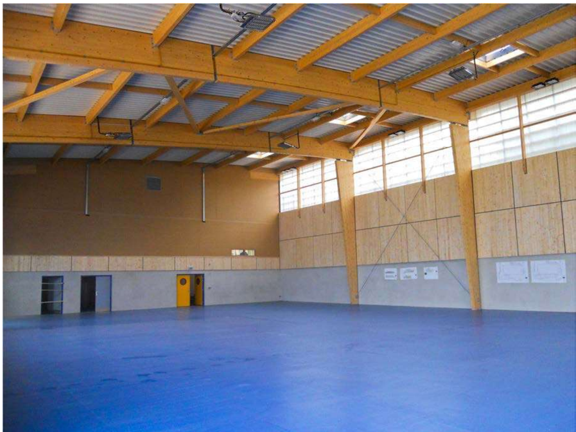
Orsay (France) Glulam structure with Résix® connections
