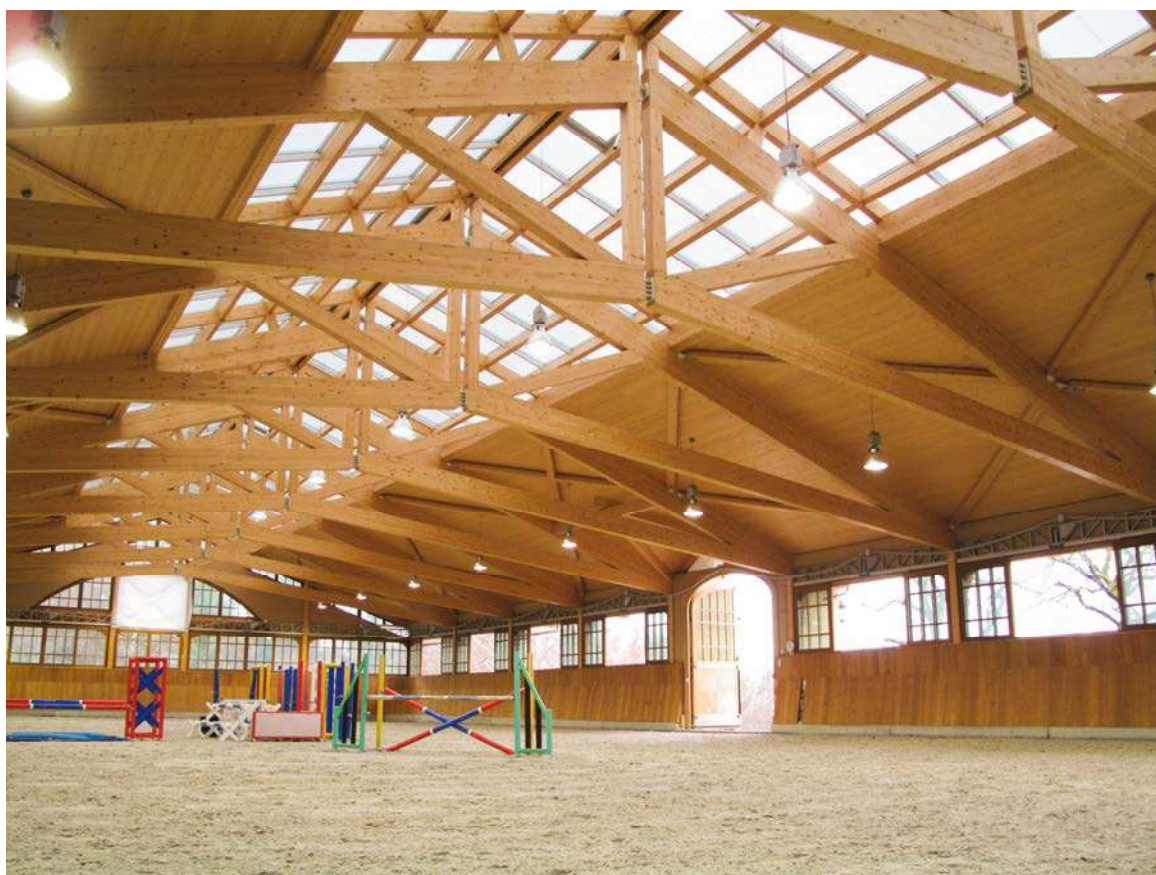
Genolier (Switzerland) Arena Glulam structure with Résix® connections
