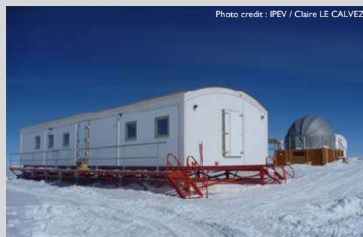
Antarctica Concordia station Sapisol® in floor, wall and roof Altitude 3000m
