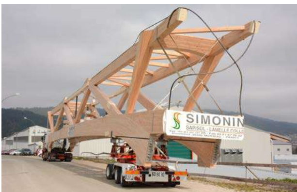
Logistics : road/sea/air Transport of 40m long bridge
