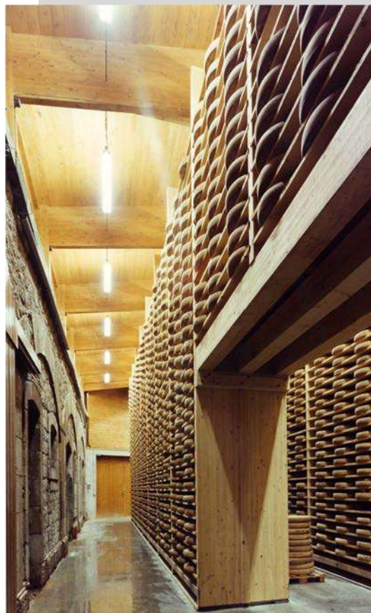
Granges-Narboz (France) Cheese maturing facility Sapisol® roofing
