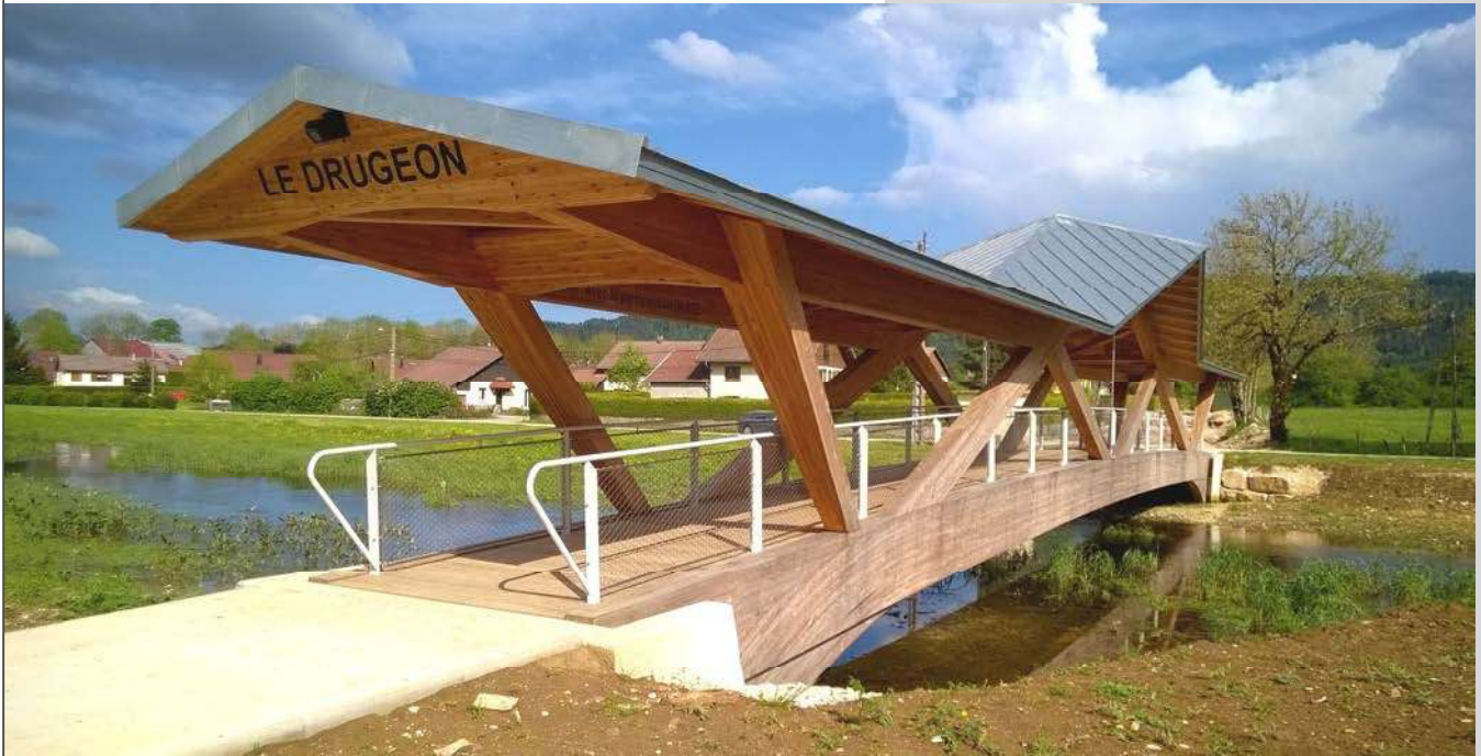
Bouverans (France) Pedestrian bridge (high voltage cable crossing) Larch structure with Résix® connections
