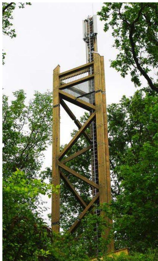
Valmondois (France) Antenna structure Glulam structure with Résix® connections 25m high
