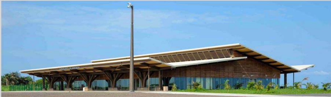
Annobon island (Equatorial Guinea) Airport Terminal Glulam structure with Résix® connections Sapisol® roofing with special acoustic profile
