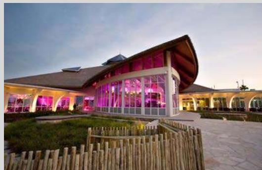
Doha - Banana Island (Qatar) Wellness center Glulam beams with Résix® connections 48 m long Sapisol sandwich panel
