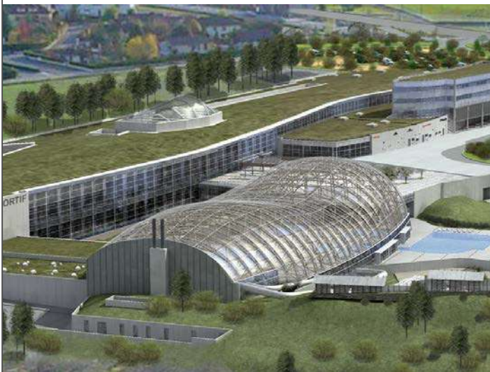
Green roof on glulam structure Wooden space frame with ETFE roofing in Aquatic Parc
