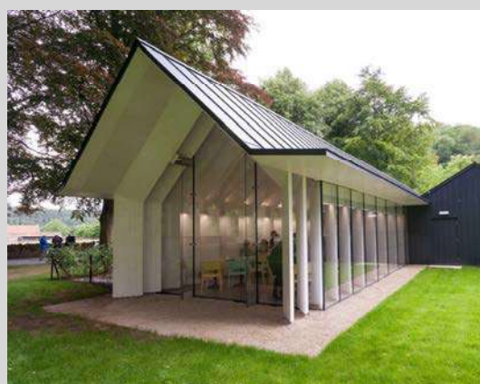
Helmsley (United Kingdom) Rievaulx Abbey Spruce glulam beams with Résix® connections
